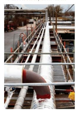
time and costs. The lack of spacers and "unforeseen" gaps minimizes heat losses and the risk of personal injuries due to hot spots on the cladding. Pipe wraps (mats) are tailored to the corresponding length of the pipe circumference on site and are fastened with clamps.
