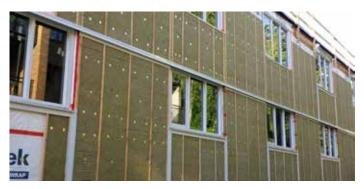
Example of insulation retained by mechanically attached impaling pins between vertical wood framing (adhesive stick-pins are not considered a long-term support strategy).
