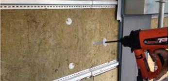
Example of plastic fuel-cell actuated insulation fasteners installed after insulation and girt system is installed to retain the insulation.
