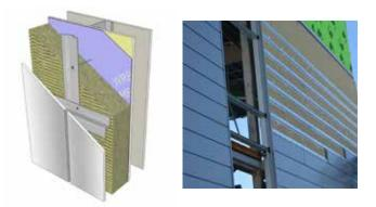
Long screws through horizontal metal hat tracks and rigid ROCKWOOL COMFORTBOARD $^{\sim}$  insulation on a commercial building project.
