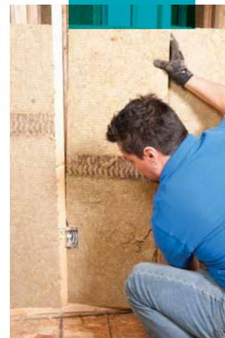
ROCKWOOL cuts quickly and accurately with a serrated knife, such as a bread knife, so you can easily achieve optimal fit around pipes, electrical boxes, wiring, ductwork and between studs and joists that are less than a standard width.
