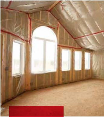
ROCKWOOL COMFORTBATT® is a semi-rigid batt insulation designed specifically for exterior wood and steel stud applications in residential and commercial construction. Made from natural stone and recycled slag, ROCKWOOL stone wool is a high-density insulation that will fit snugly into wall cavities and will not slump over time. It also adds superior acoustical performance to wall assemblies and floors and can be used in acoustic applications required by building code.
